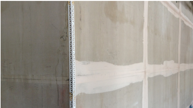
Rebated fibre cement flushed and beaded ready for rendering
