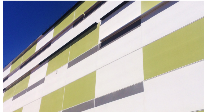
Acrylic render system applied to panels
