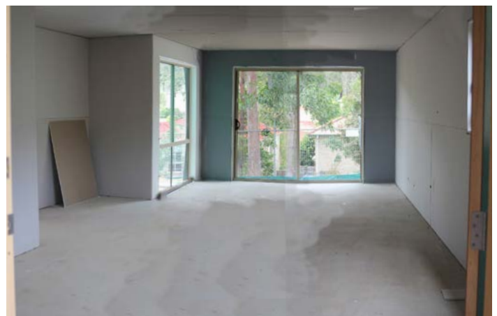
Interior EPS Panels with screw fixed plasterboard
