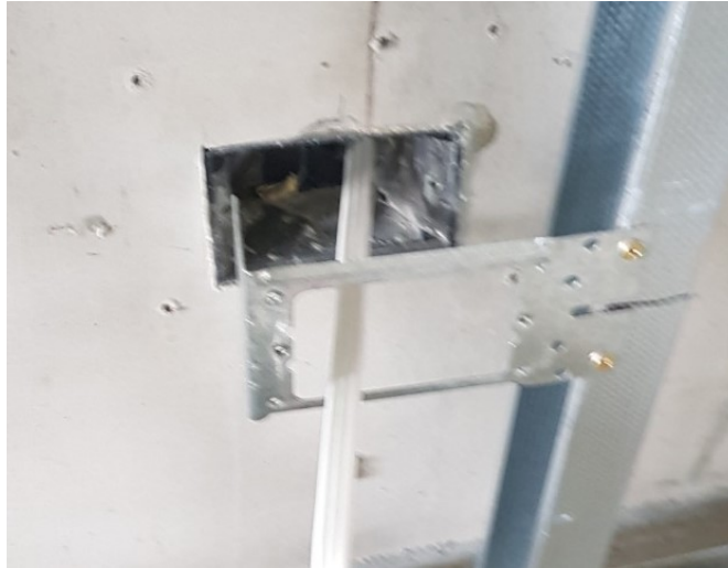
Installation of wall box in fibre cement panels
