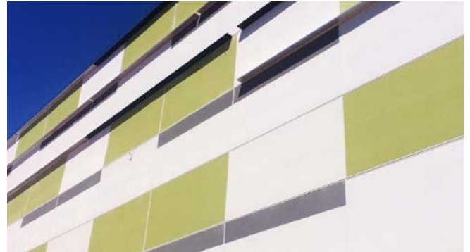
Acrylic render system applied to panels
