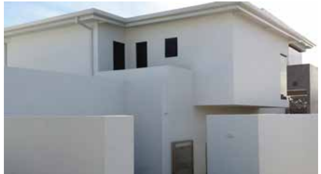
3. EPS panels with acrylic textured render system
