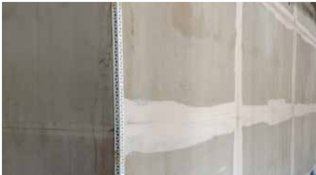
2. Rebated FC flushed and beaded ready for rendering
