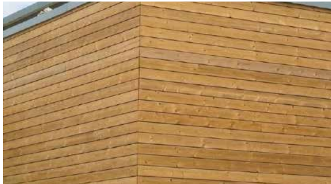
1. Cladding fixed to FormPro® wall system
