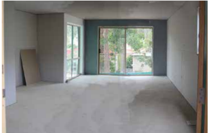
Interior EPS Panels with screw fixed plasterboard
