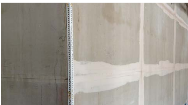
Rebated FC flushed and beaded ready for rendering
