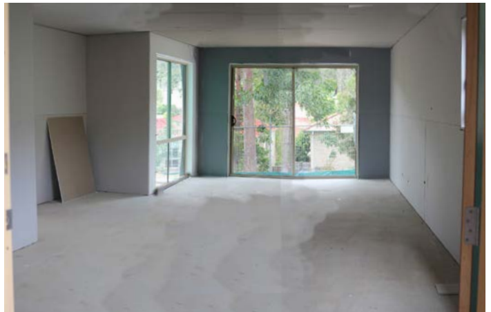
Interior EPS Panels with screw fixed plasterboard
