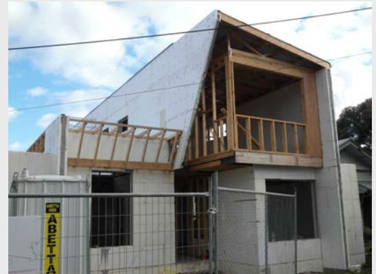
Mark & Ambia's home in construction
