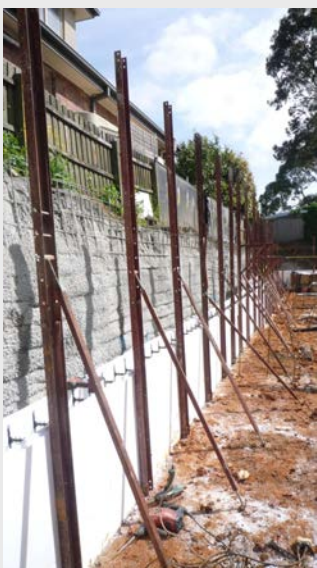
Bracing basement walls, East Brighton
