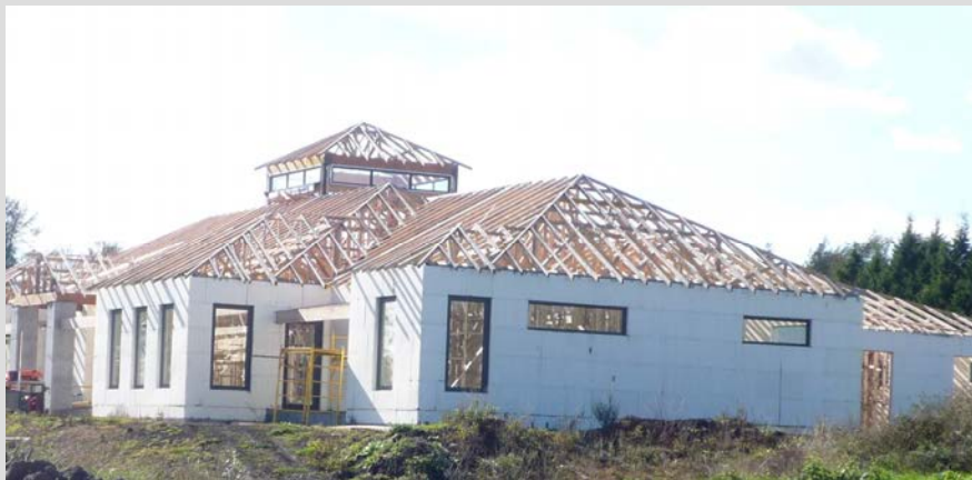
Sue & Sam's home structure completed by Formcraft Vic
