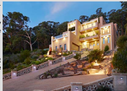
Exterior of completed home by night
